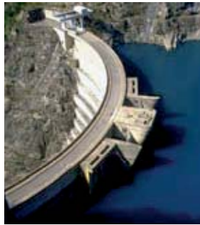
Reservoir (level control)
