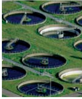
Wastewater treatment plants (overflow protection)
