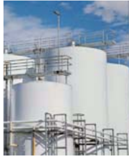
Tank farms (level monitoring)
